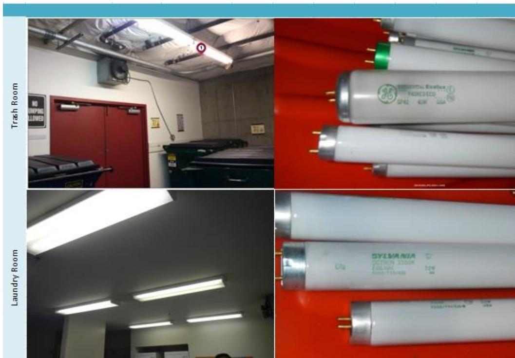
Figure 9. Energy and lighting audit
