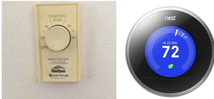
Figure 11 - Existing thermostat (Left) & “Smart” Thermostat (Right)
